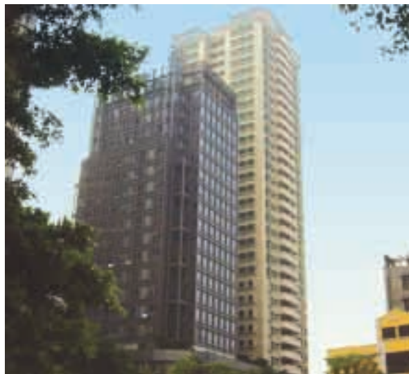
Project at 17-43 Beijing Nan Road, Guangzhou, Guangdong Province, PRC
