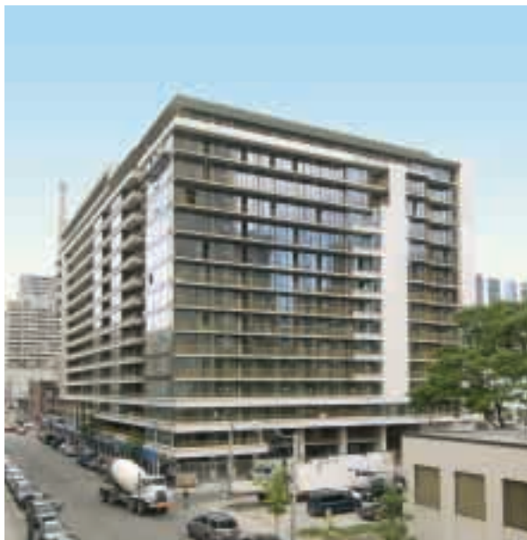
One City Hall (Phase I) at South-West Corner of Bay Street and Dundas Street West, Toronto, Ontario, Canada developed by Hon Kwok Land Investment Company, Limited
