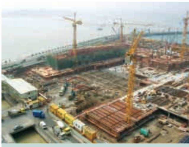
Piling, pile caps and basement construction work at MGM Grand Macau at Nam Van, Macau undertaken by Chinney Timwill Construction (Macau) Co., Ltd.
