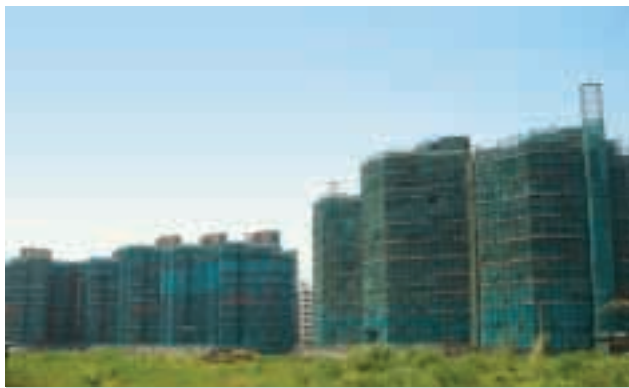
Construction site of Long Dong Cun at Guangshan Road Western, Tianhe District, Guangzhou, Guangdong Province, PRC held by Hon Kwok Land Investment Company, Limited
